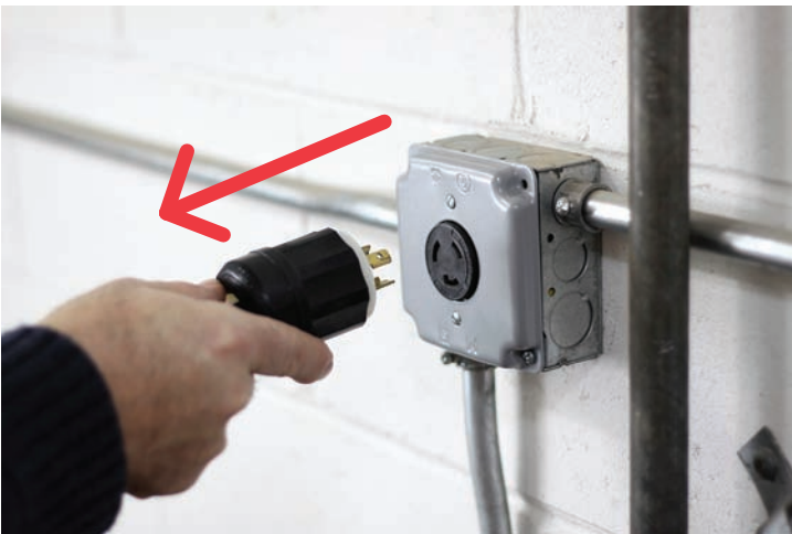
3 Disconnect the power tool from the power source before changing the saw blade.
